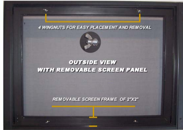
SAMPLE OF SCREEN WALL - POOL ENCLOSURE
